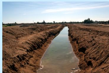
Unlined drainage canals, sandy gravelly soils underlined by poorly permeable bedrock enhanced drainage problems.
